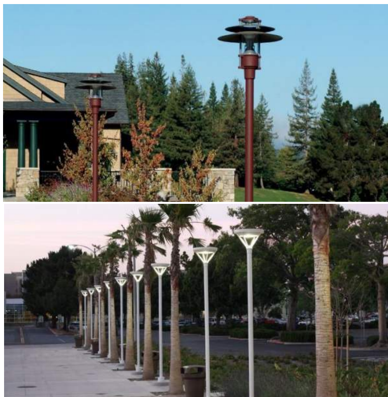
Figure 5.0-12, Post Lighting Examples
