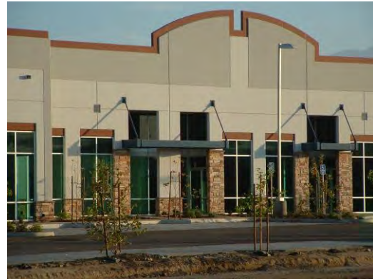
Roofs and Parapet
