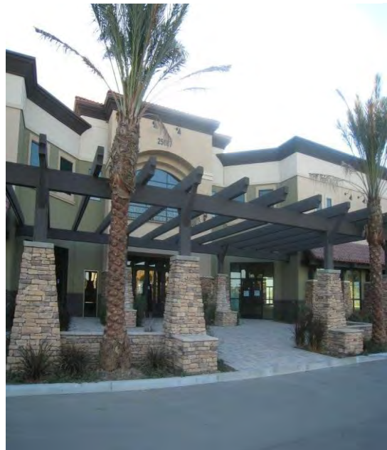
Building Entrances and Access Points
