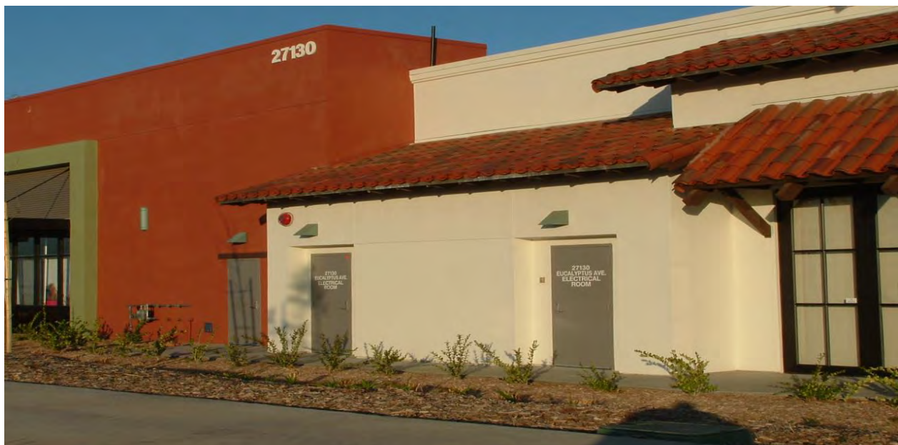
Built in Utility Equipment Room
