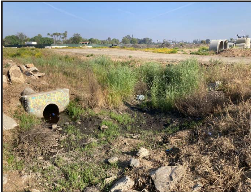
PHOTOGRAPH 8 - Northward View of Ellis Avenue Roadside Drainage Ditch Culvert.
