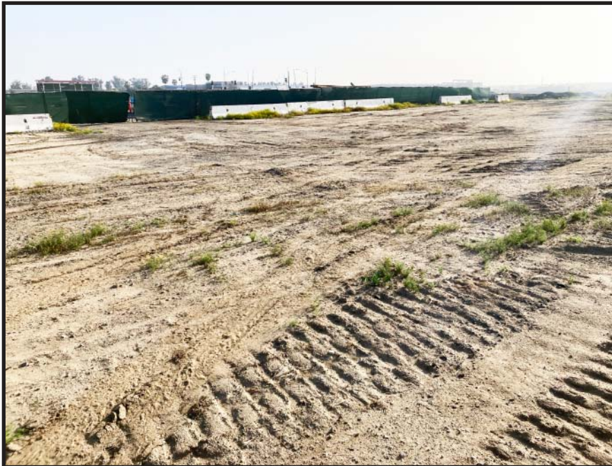
PHOTOGRAPH 2 - Northeast View of Project Site.
