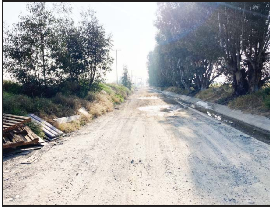
PHOTOGRAPH 7 - Eastward View of Ellis Avenue.
