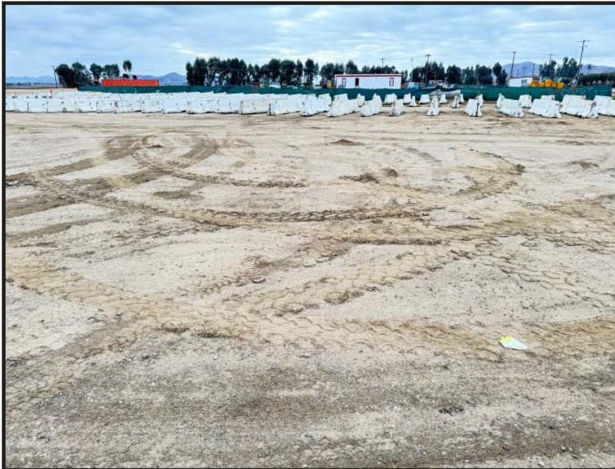
PHOTOGRAPH 8 - Southward view of Project Site from Case Road and Goetz Road intersection.
