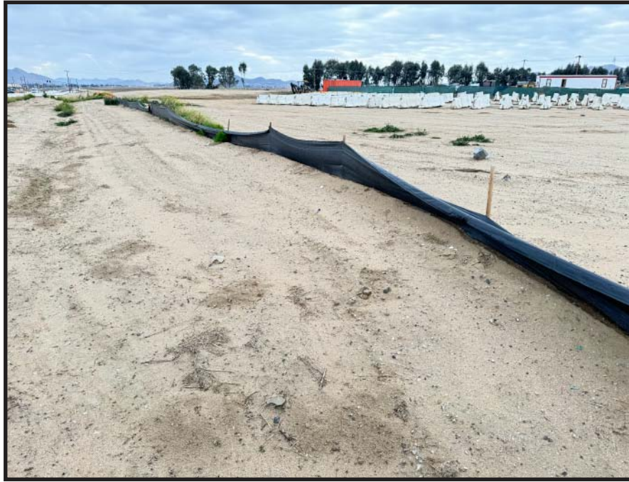
PHOTOGRAPH 7 - Southeast view of Project Site from Case Road and Goetz Road intersection.
