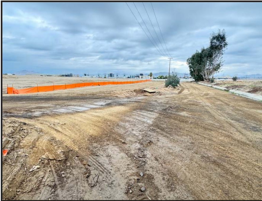
PHOTOGRAPH 4 - Eastward View of Project Site and Ellis Avenue.
