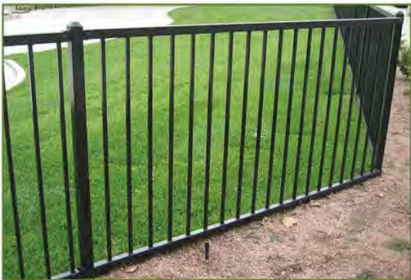
Community Prefabricated Tubular Steel View Fence
