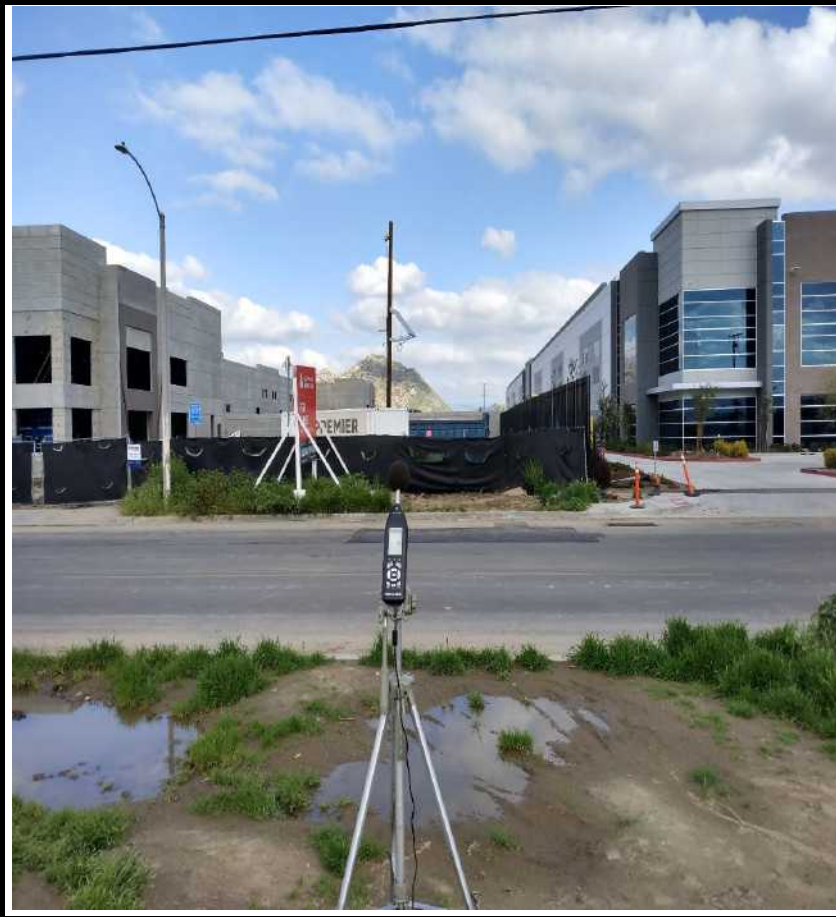
STNM5 looking E across Wilson Avenue. Building at 3125 Wilson Avenue on right of image & warehouse under construction on left of image.
