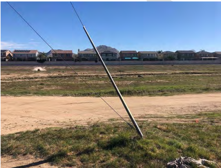
Photograph 6. Perris Valley Storm Drain - Facing East.
