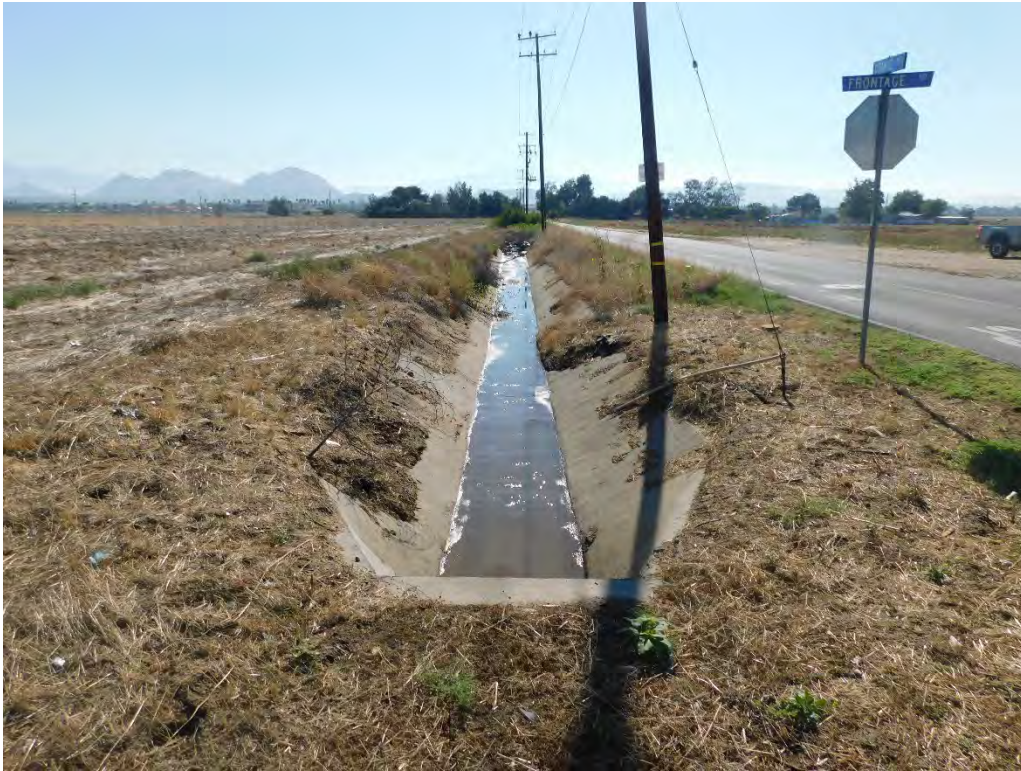
Photograph 9: From inside Drainage 2 looking east at its entry to the project site at the intersection of Orange Avenue and Frontage Road along the western boundary.
