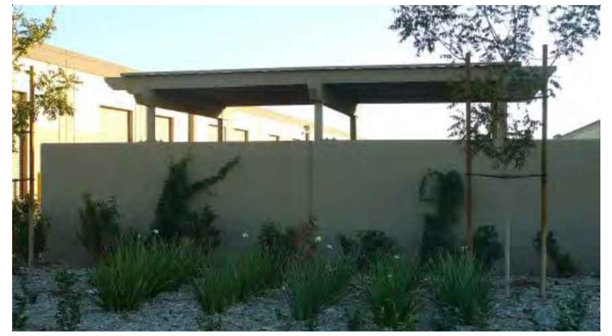
Trash enclosure with overhead trellis treatment
