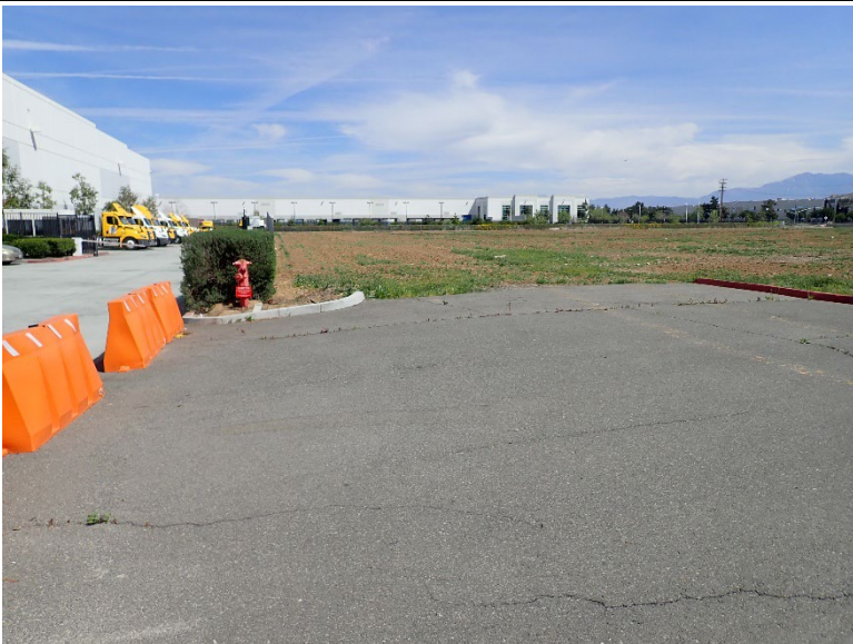
Photo 3: View north along west property boundary at adjacent development, public improvement driveway & disked site. 4/12/2025
