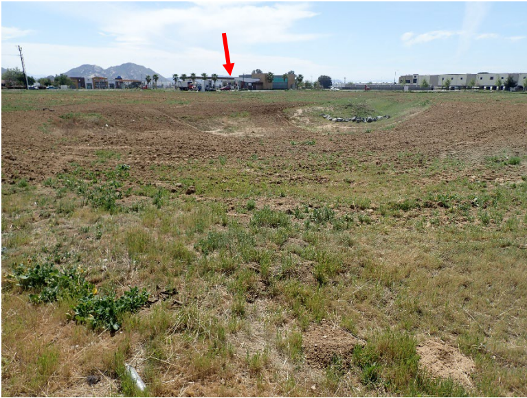
Photo 9: View east across disked site, detention basin, 7-Eleven gas station (arrow), and surrounding development. 4/12/2025
