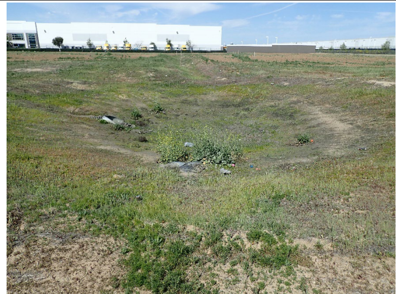
Photo 8: View west at constructed stormwater detention basin/swale, ruderal non-native vegetation, & adjacent development. 4/12/2025
