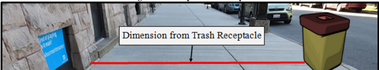
Sidewalk Picture Showing Trash Receptacle in Compliance with Clearance
