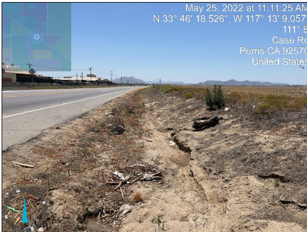
Unvegetated streambed ditch along Case Road.
