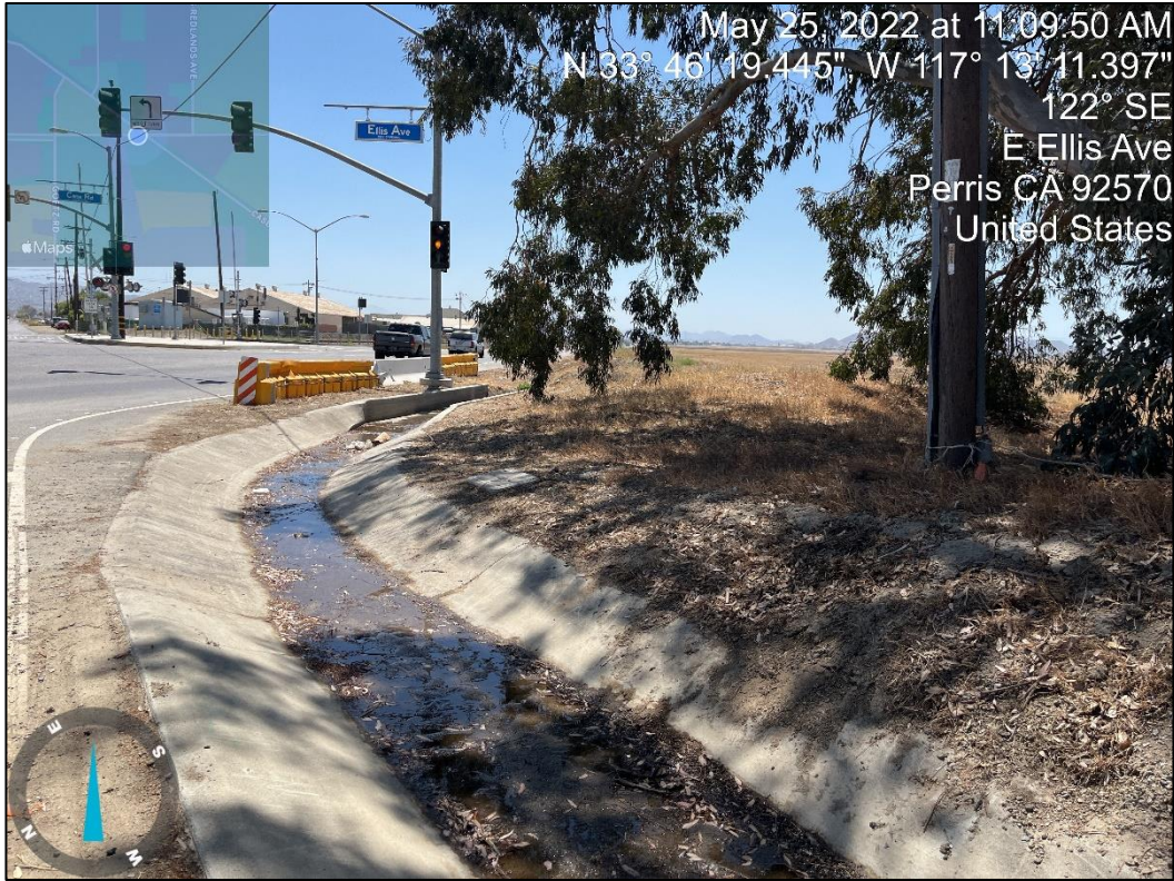
The concrete lined channel continues to Ellis Avenue and Case Road.
