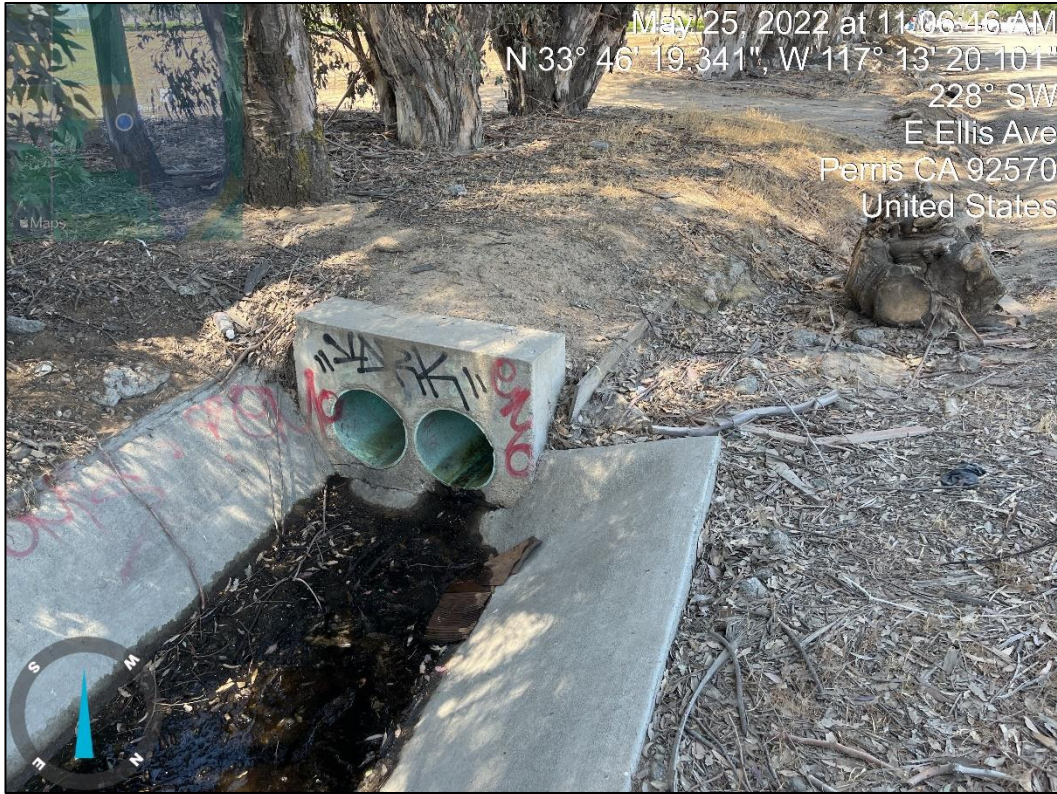
Beginning of concrete lined channel along Ellis Avenue.
