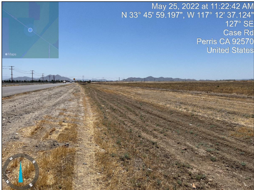
Ditch A along Case Road appears to be maintained.
