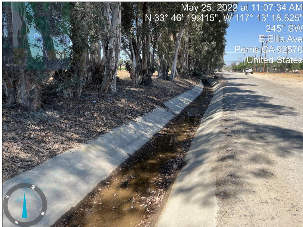
Concrete lined channel along Ellis Avenue.
