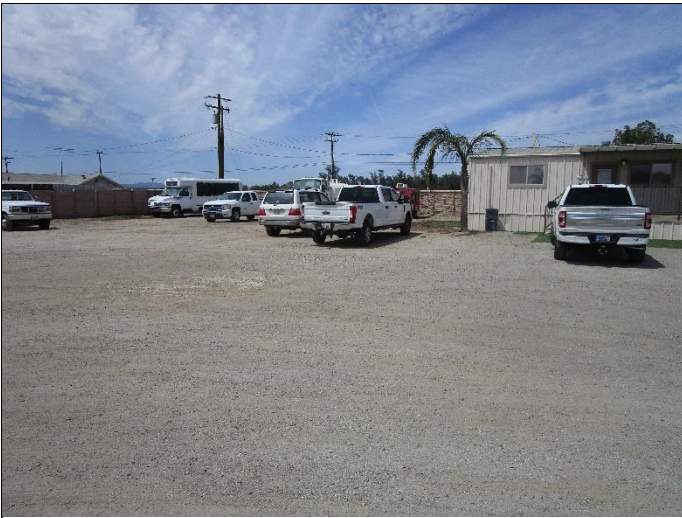
3. View of location of septic system tank leach field.
