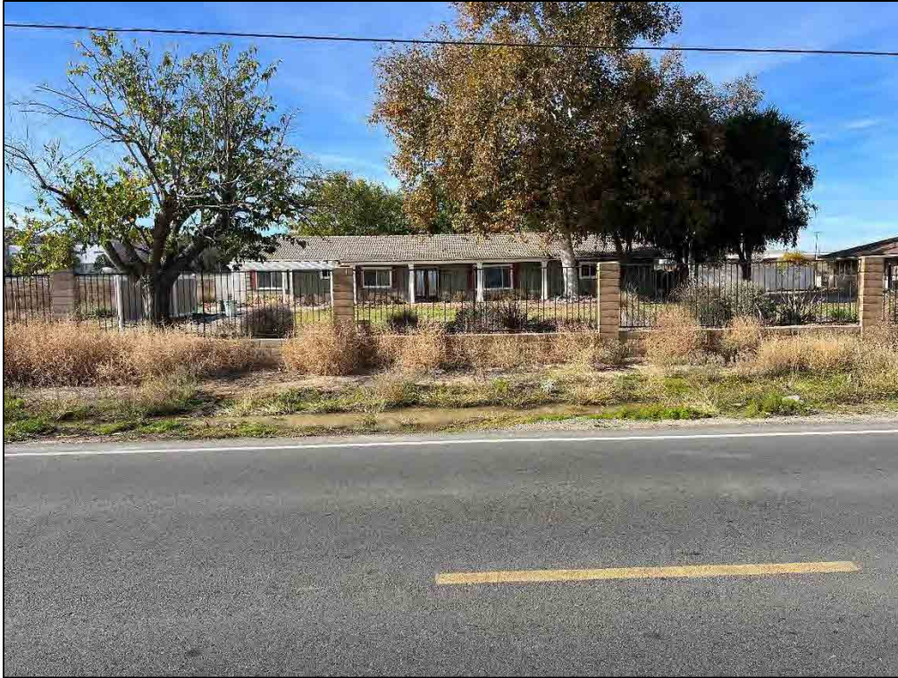
Photo 50. View of the residence from Indian Avenue.
