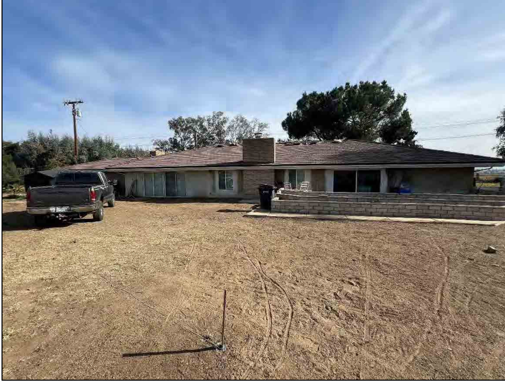
Photo 37. View of the west (rear) elevation.
