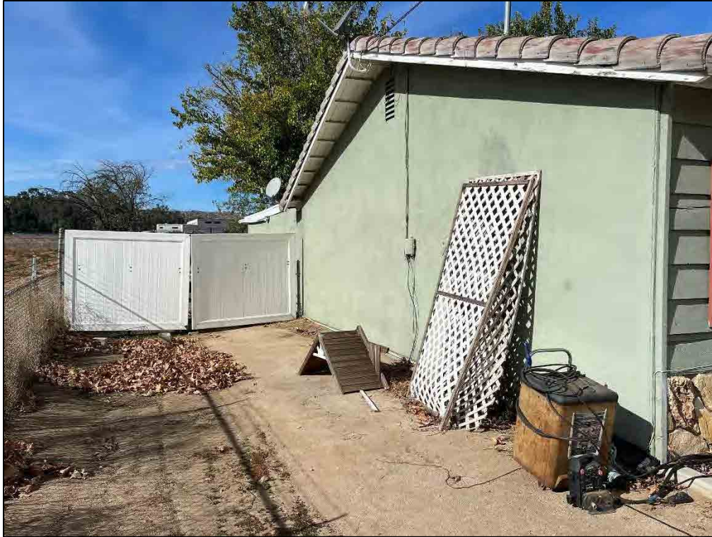
Photo 52. View of the south elevation.
