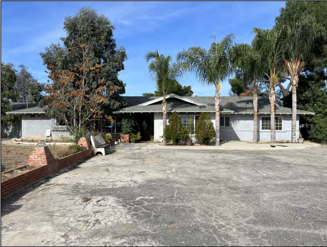
Figure 6. View west of 2411 Indian Avenue.
