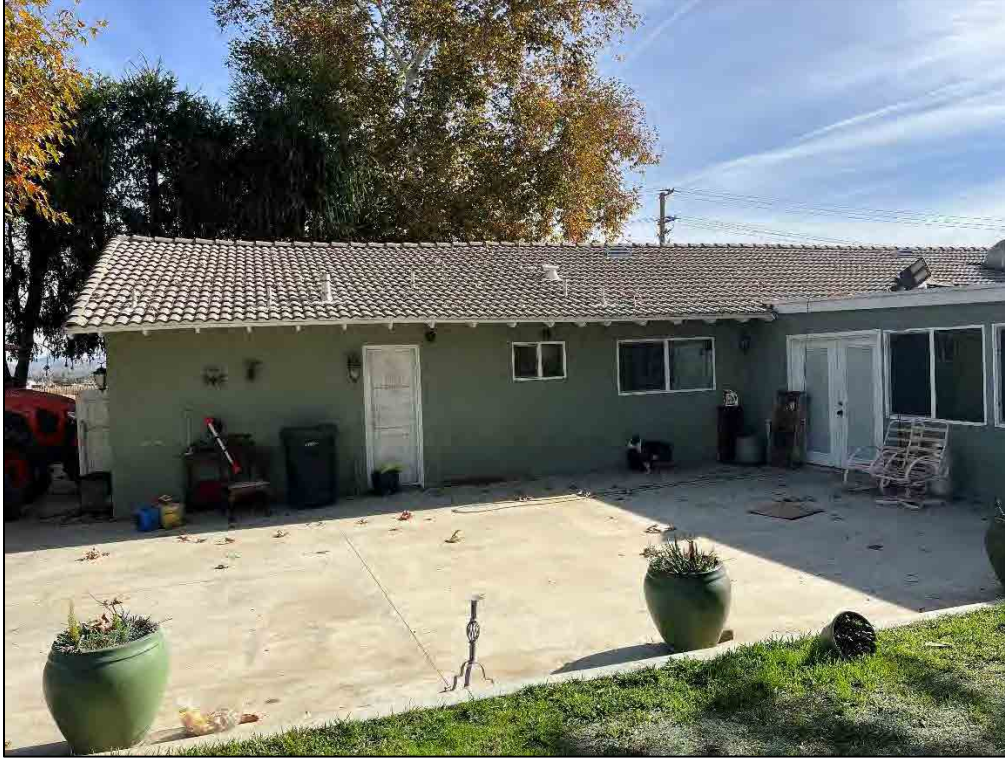
Photo 58. View of the rear elevation.
