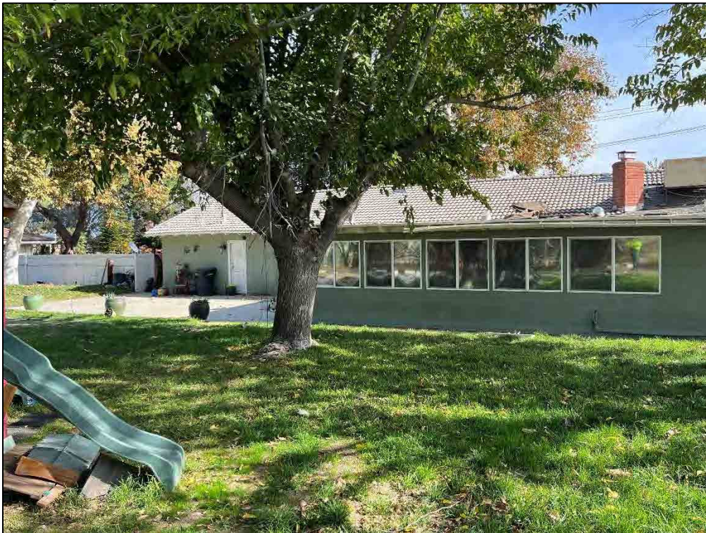
Photo 55. View of the rear elevation.
