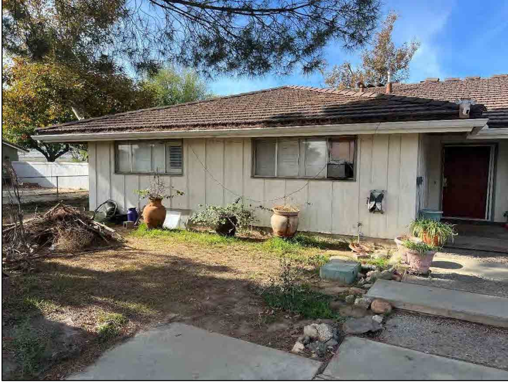
Photo 31. View of the front elevation.
