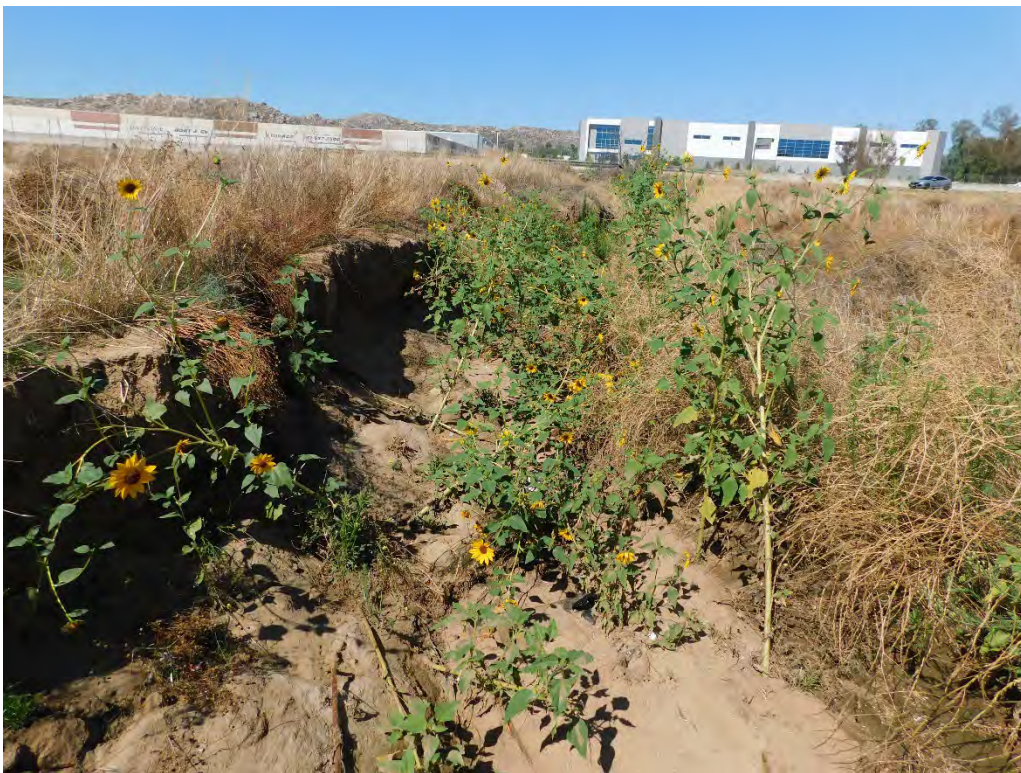
Photograph 4: From the middle of Drainage 1, looking west.
