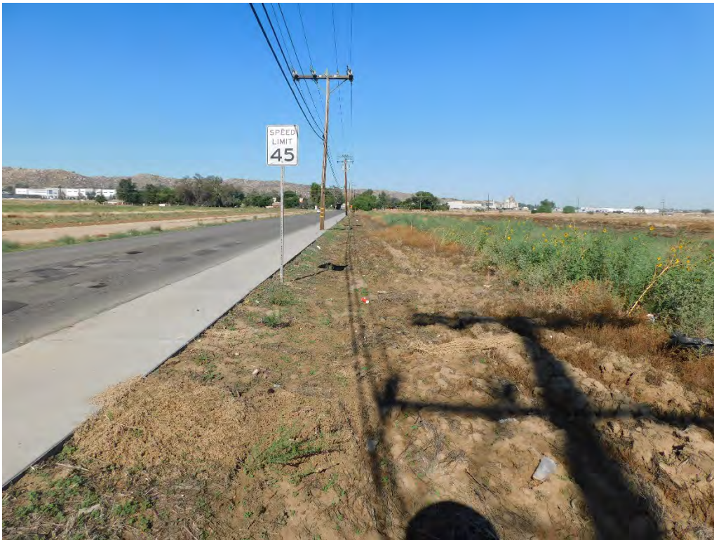
Photograph 10: Looking west at the road side ditch along Orange Avenue between Barnett Avenue and Indian Avenue.
