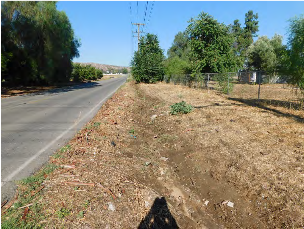
Photograph 9: From Indian Avenue looking west at the road side ditch along Orange Avenue.
