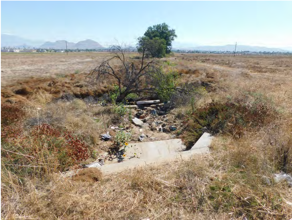
Photograph 1: From the top of the culvert under I-215, looking east at the beginning of Drainage 1 on the western boundary of the project site.
