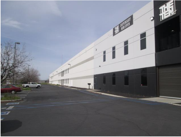
1. Southern portion of the Site.
