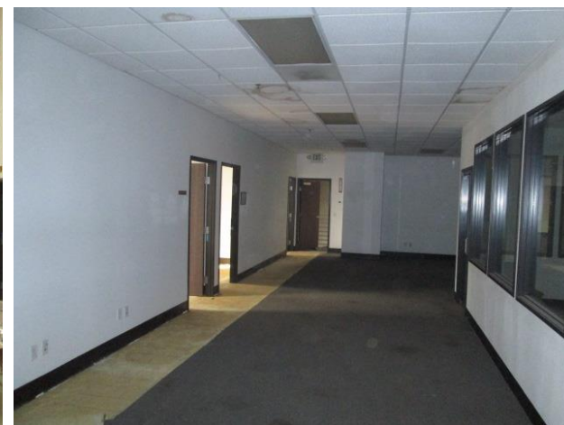
12. Western mezzanine level.
