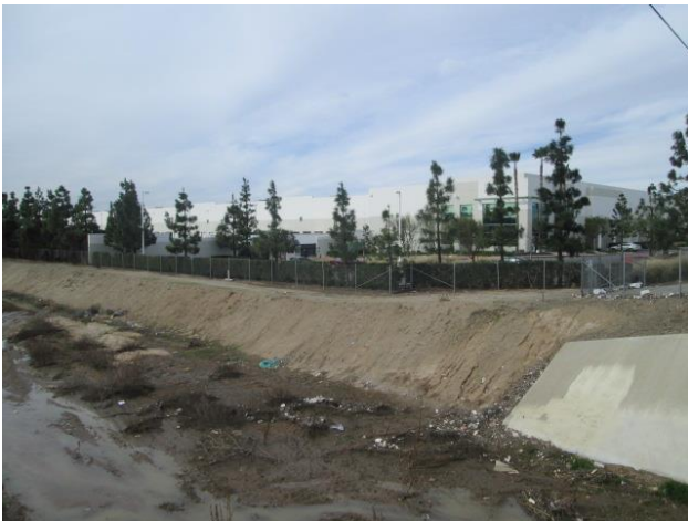
16. Northern adjacent commercial property.
