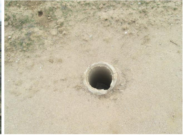
9. Typical utility feature.
