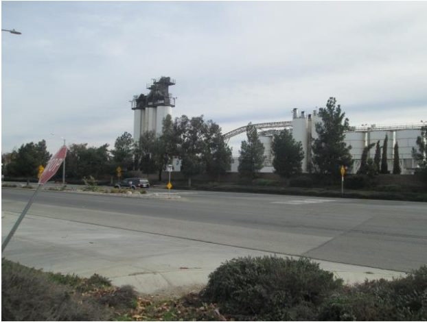
13. Southern adjacent Harley Knox Boulevard and asphalt plant.
