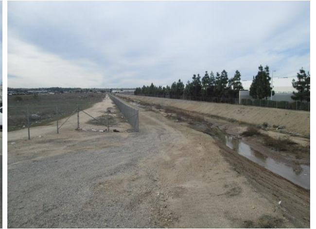
15. Northern adjacent East Oleander Avenue (unimproved) and drainage.
