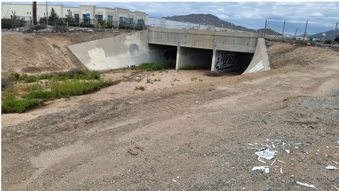
Photograph 6 NE Corner. Looking East at Flood Control Channel Box Under Indian Avenue
