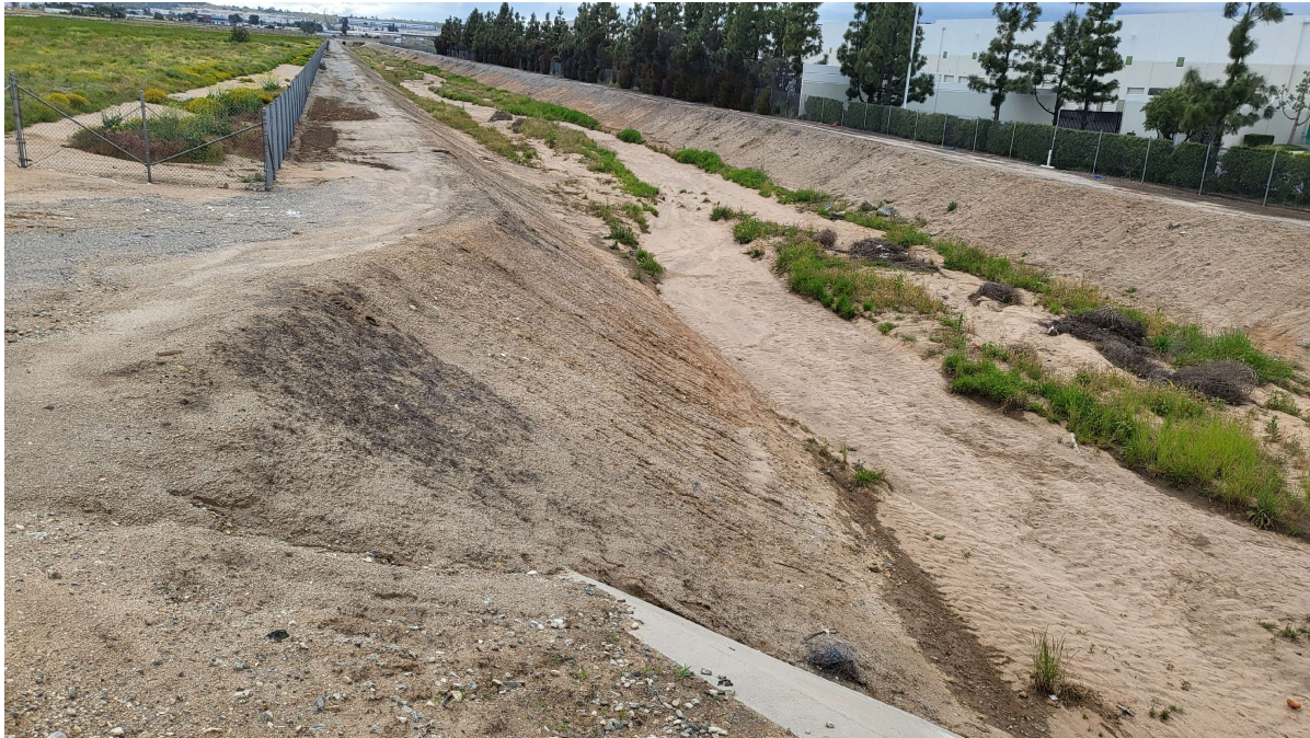
Photograph 5 NE Corner. Looking West. Developed Flood Control Channel (maintained)
