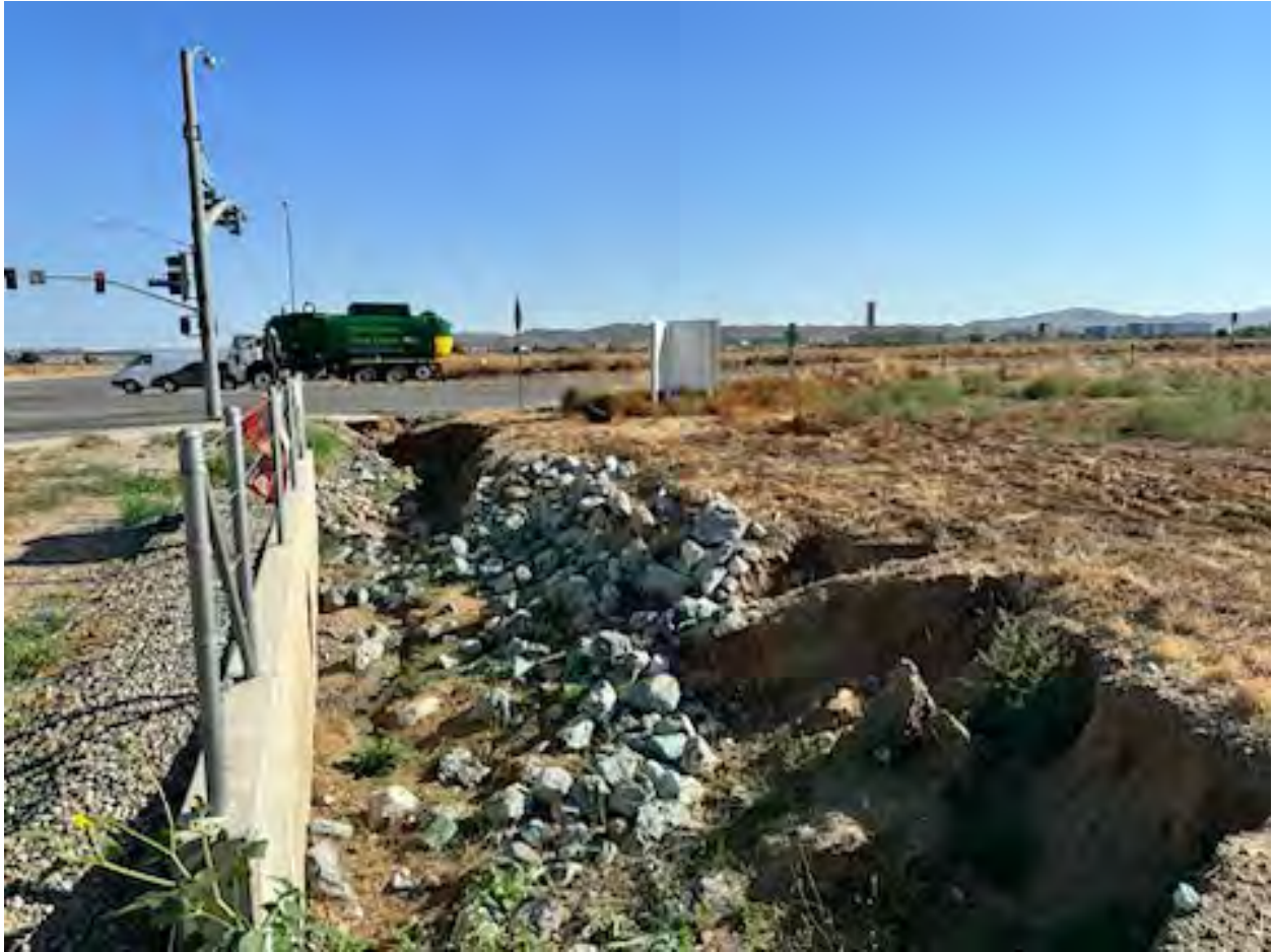
Storm drain located in the southeast corner of the site.
