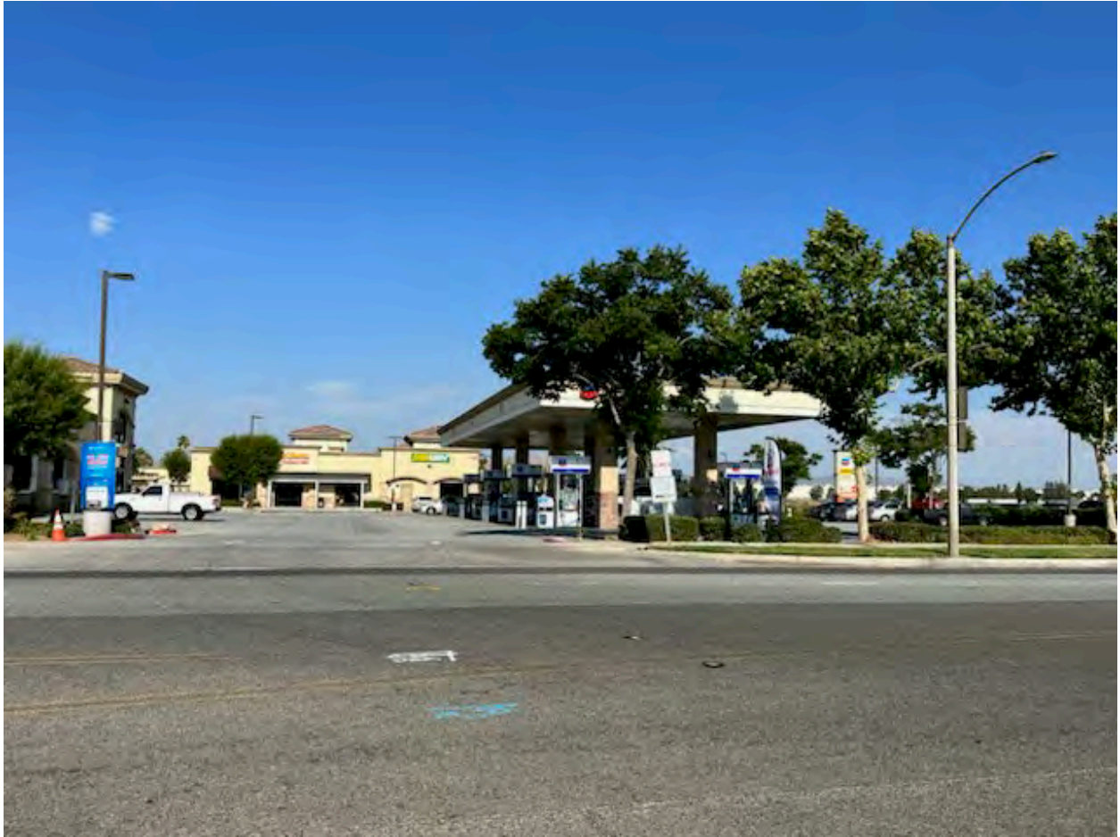
Chevron Gasoline Station located east of the site beyond North Webster Avenue.
