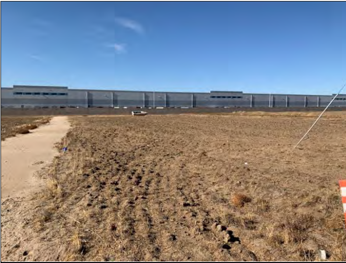
19. The adjoining properties to the west, view facing south.
