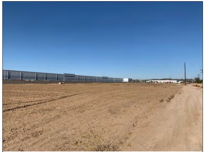
16. Subject property from the north central boundary, view facing west.
