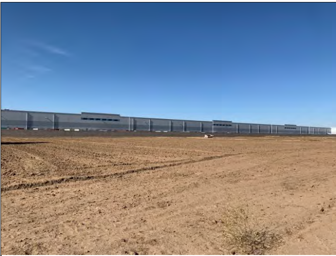
15. Subject property from the north central boundary, view facing southwest.
