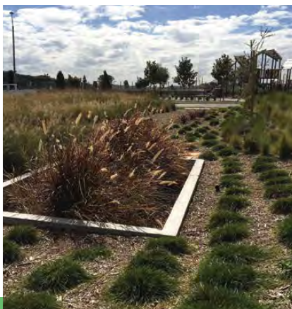
Open Top Planter - Filterra Bioscape
