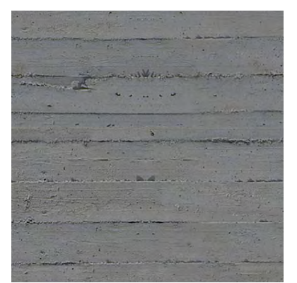
14 Board Formed Concrete
