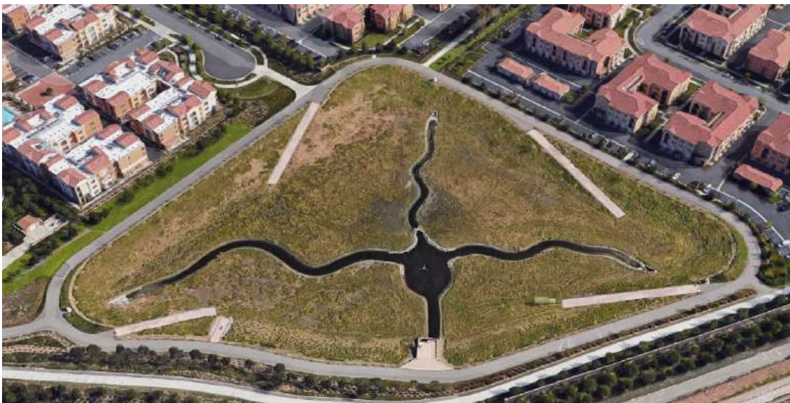
Figure A: Detention Basin BMP
