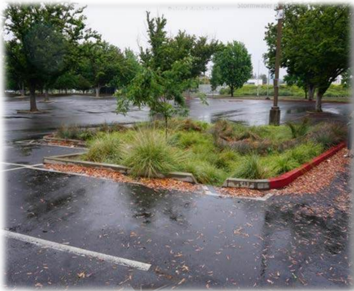
Figure A: CA State University-Sacramento Bioretention BMP
