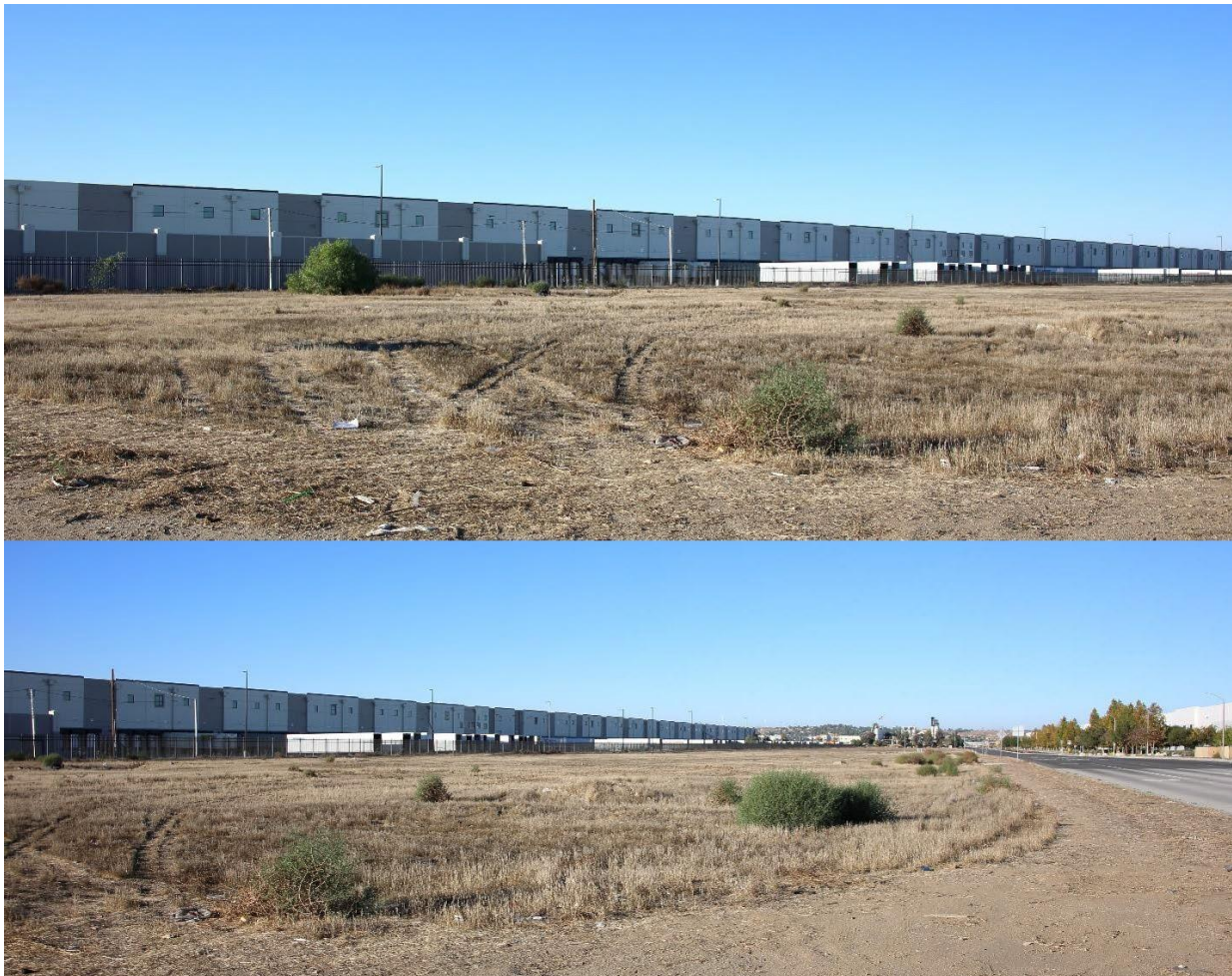
Photos 1 and 2. Views of the project site on 21 November 2021. Photos by Noriko Smallwood.
