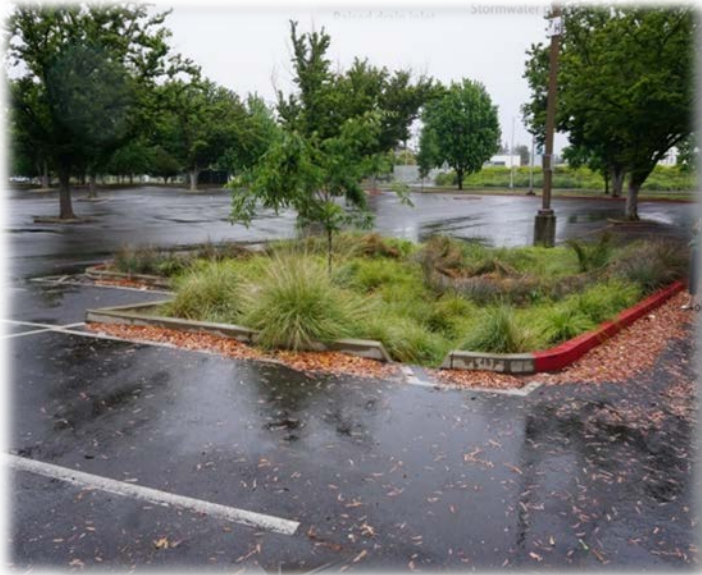
Figure A: CA State University-Sacramento Bioretention BMP
