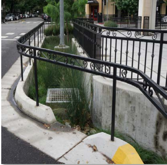
Figure A: Urban Infiltration Trench BMP
