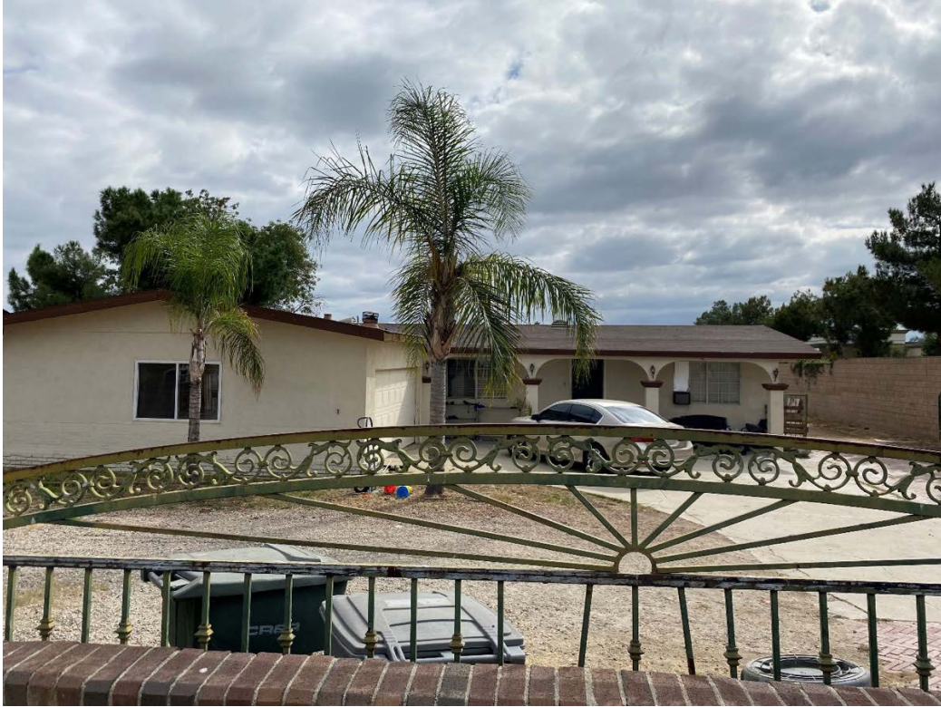
Photo 1 - Front of residential structure; East view.
