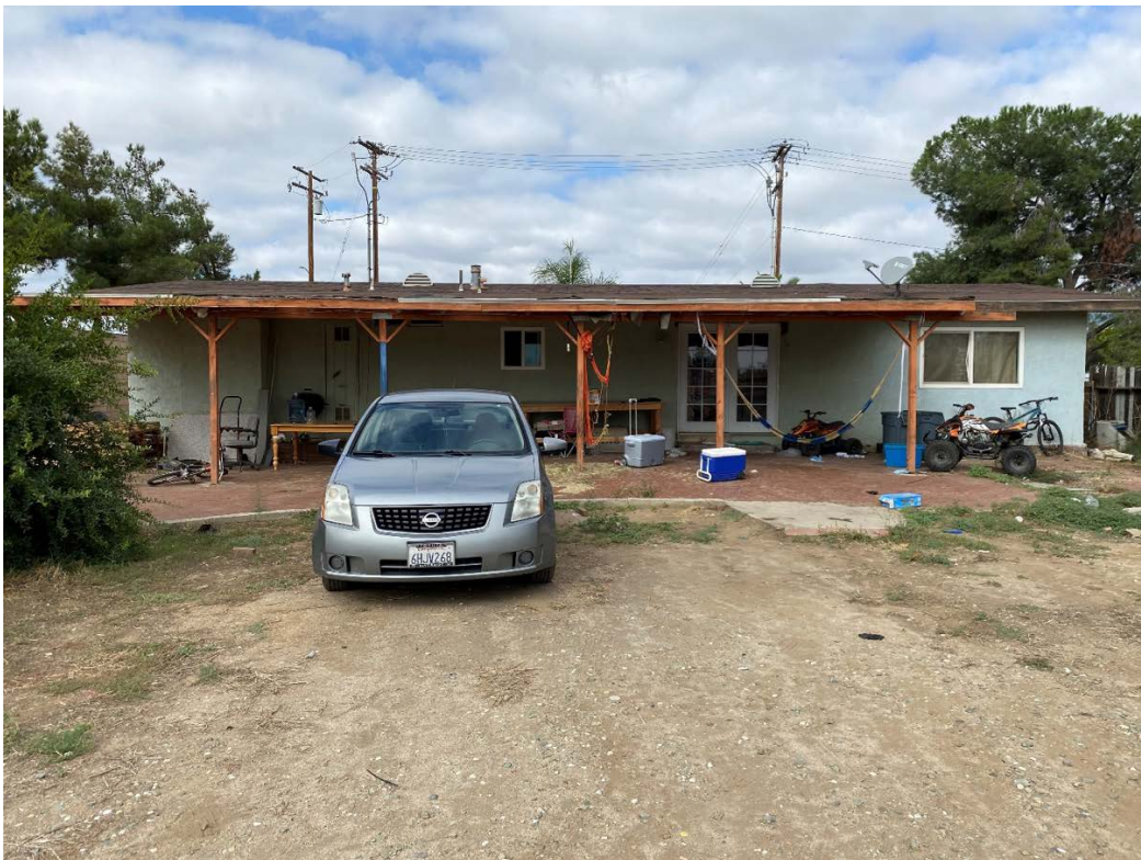
Photo 2 - Rear of residential structure; West view.
