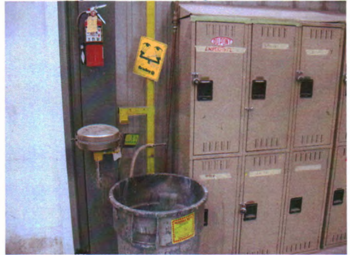
Emergency equipment access blocked
