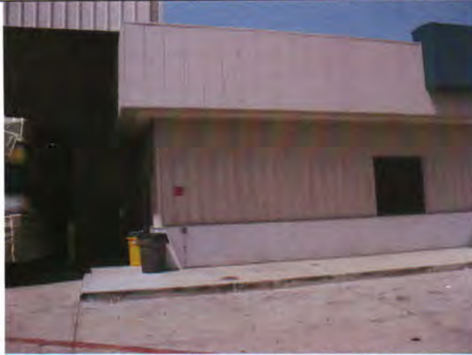
Propane emergency shut off switch
