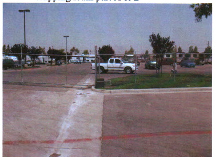
Storm water discharge violation
