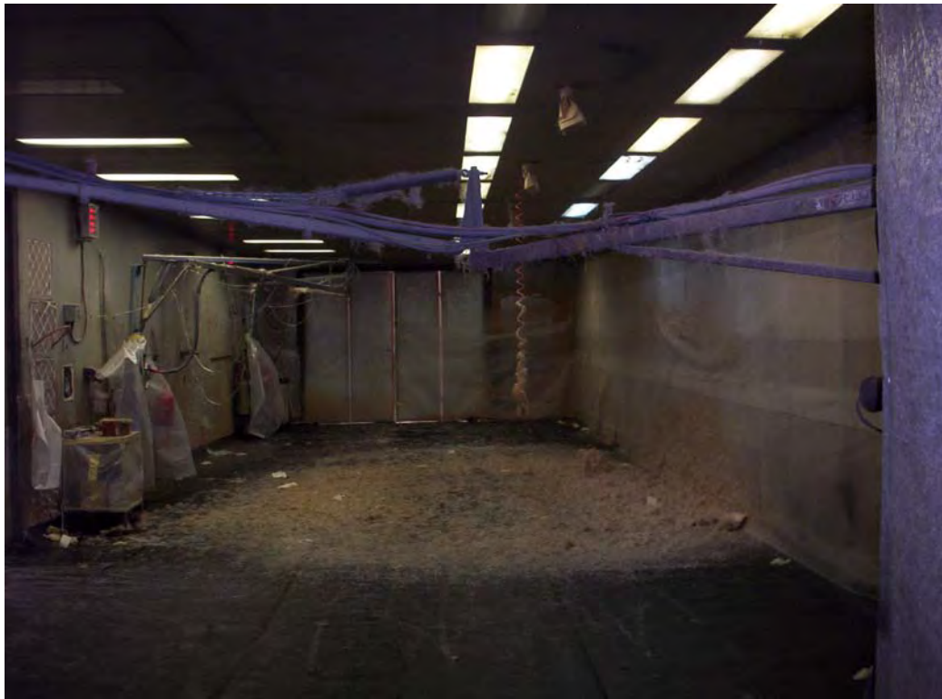
Photo #4: Resin application area within Building 3 (3411 N. Perris Boulevard).
