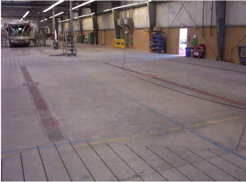
Photo #15: Rain test area within Building 5.
