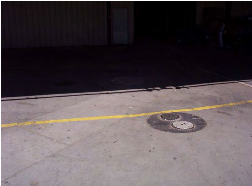
Photo #6: Indicator of the 8,000-gallon gasoline UST adjacent to Building 1.
