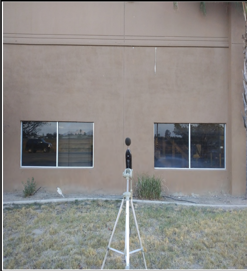
STNM5 looking S directly at the northern side of building 27271 Ethanac Road, Menifee.
