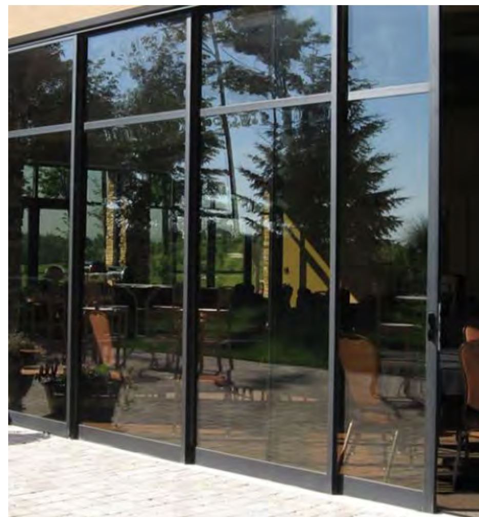
2 Storefront Storefront Glass Manufacturer: Arcadia - Color #85 Dark Bronze AB-7 Vitro Arch. Glass - 1" Clear Float Glass
