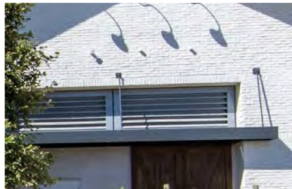
14 Wall Louvers Manufacturer: Architecture Wall Louvers Model: 4" Standard Blade Color: DE 6385 Black Bean - Semi Gloss By Dunn Edwards
