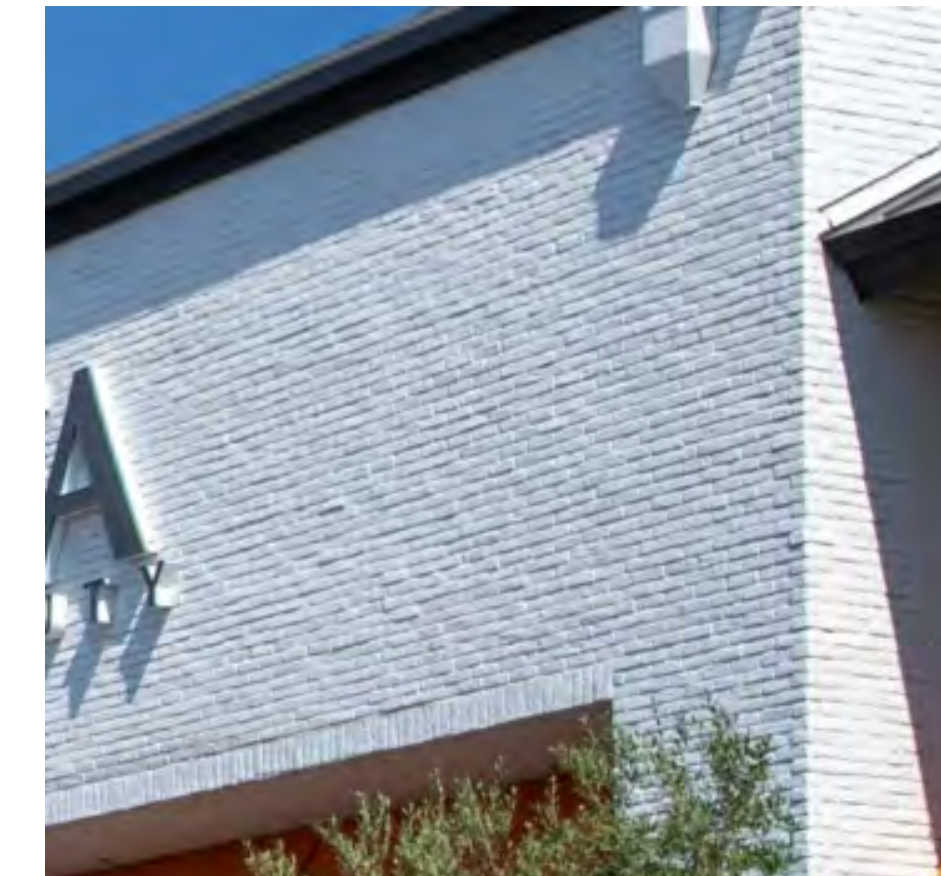
3 Brick Veneer Manufacturer: Interstate Brick Model: Thin Modular 21/4 x 8 Color: Arctic White #381 Bright White By Customs Build'g Product
