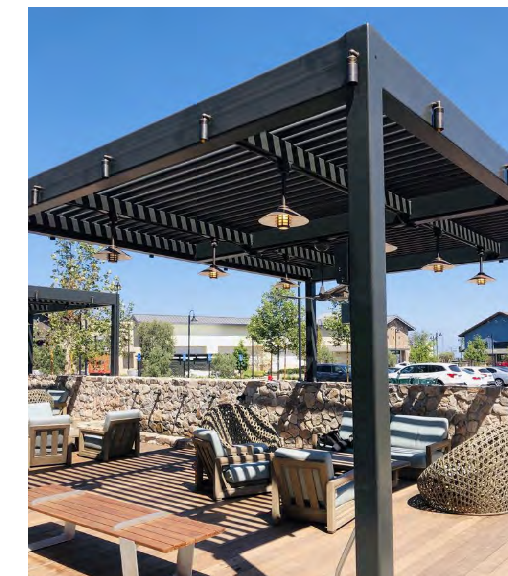
11 Metal Trellis, Post & Steel Framing Manufacturer: By General Contractor Finish: Painted Color: DE 6385 Black Bean - Semi Gloss By Dunn Edwards
