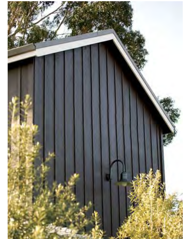
4 Batten Board Siding Manufacturer: Hardie Board Model: Hardie Plank Smooth Vertical Panels (10"x4"x5/16") w/ Trim Boards (1"x3.5") Color: Primed and Painted w/ 2-Coats Flat Acrylic Latex - Eggshell By Dunn Edwards Batten Spacing at 12" Center to Center.
