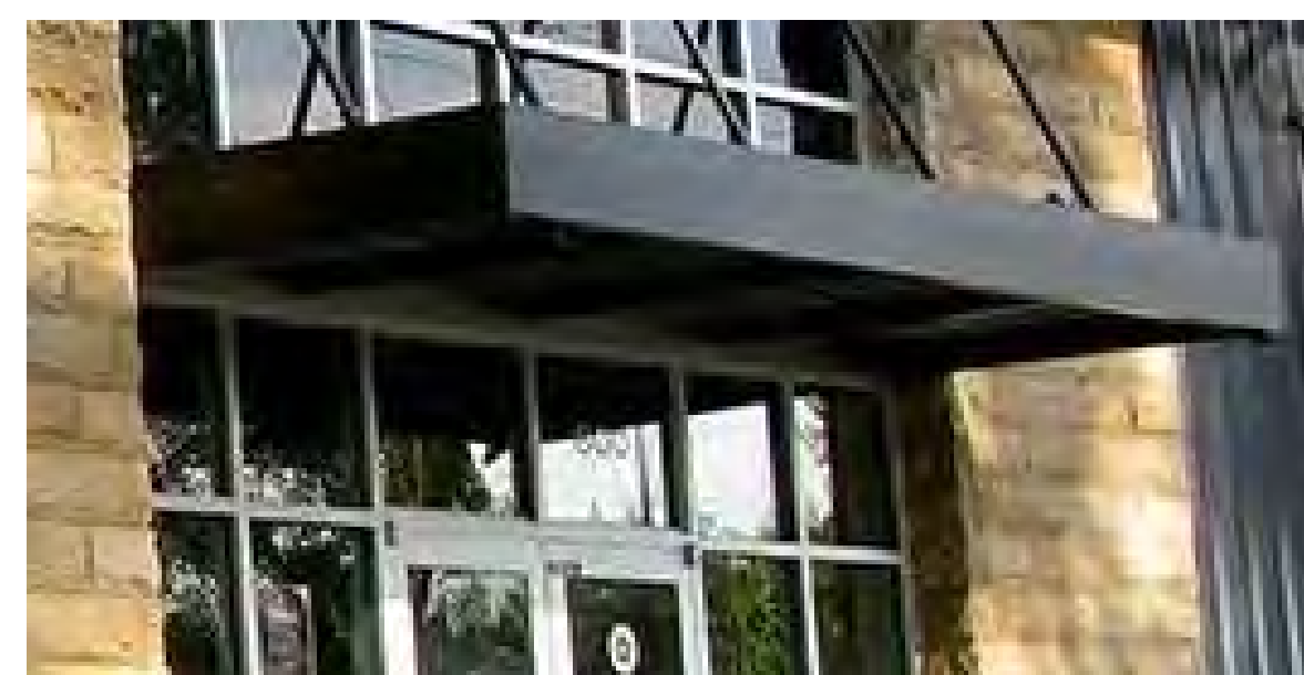
9 Metal Canopy Manufacturer: By General Contractor Finish: Painted Color: DE 6385 Black Bean - Semi Gloss By Dunn Edwards
