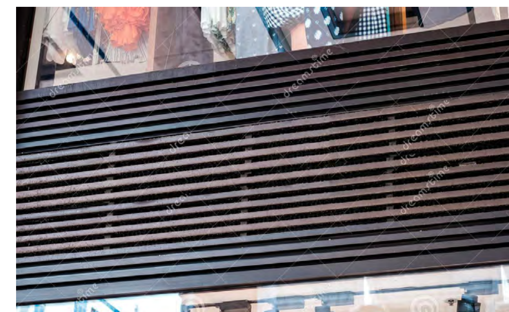
10 Metal Slats Manufacturer: By General Contractor Finish: Painted Color: DE 6385 Black Bean - Semi Gloss By Dunn Edwards
