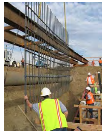
Metropolitan construction crews
