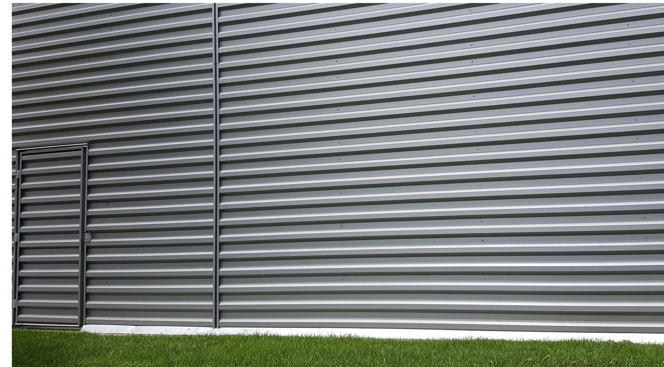
CORRUGATED METAL CLADDING BEFORE PAINT COLOR APPLIED SEE P3 FOR COLOR
