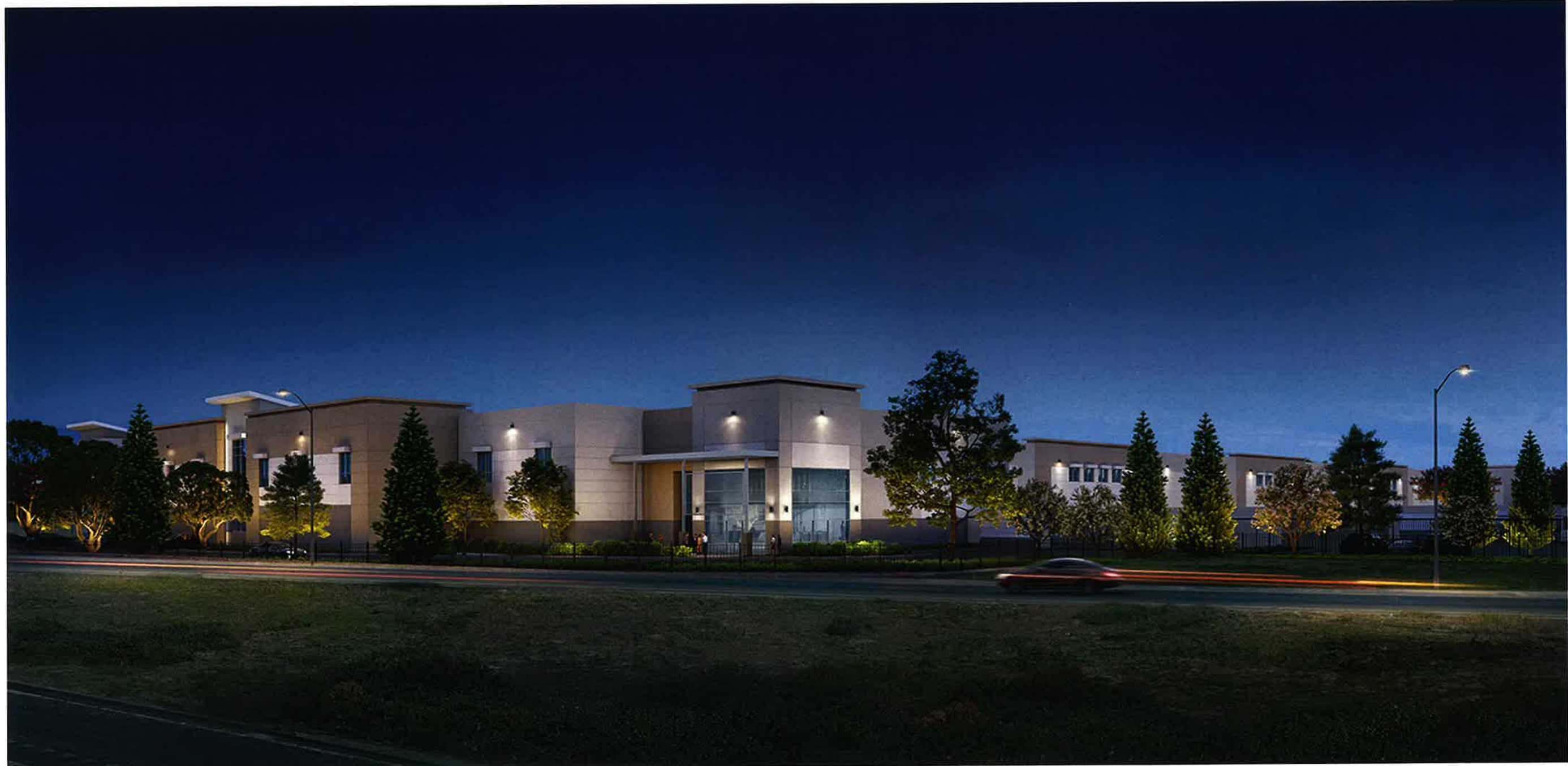
VIEW FROM FREEWAY 215 LOOKING NORTHEAST
