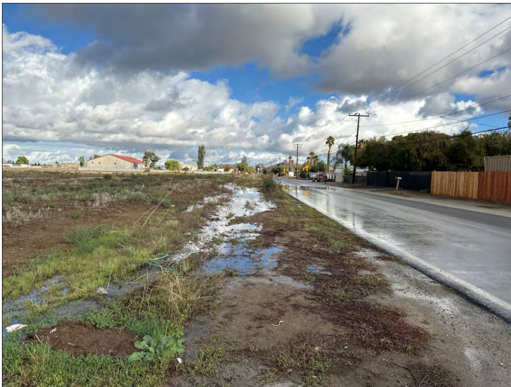
Photo 6: View of Trumble Road and western side of Project Footprint where road improvements will occur; facing north.
