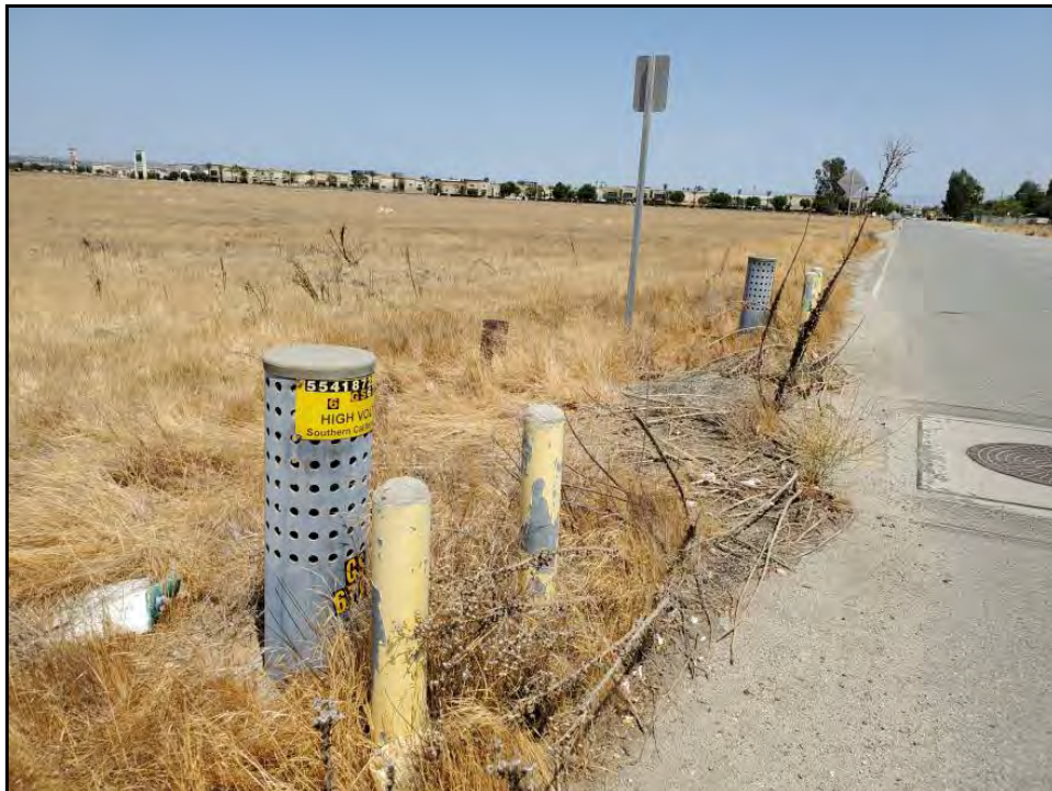
Buried power line along east boundary of the Property
