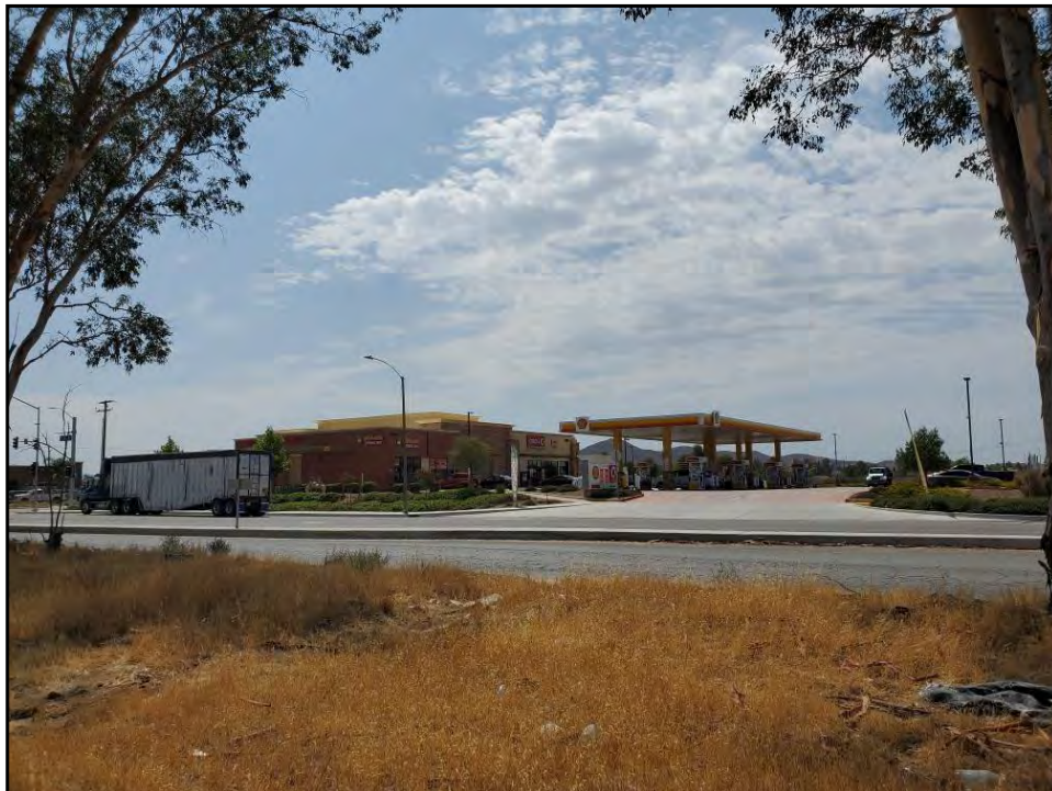
Gas station facility adjacent and south of the Property
