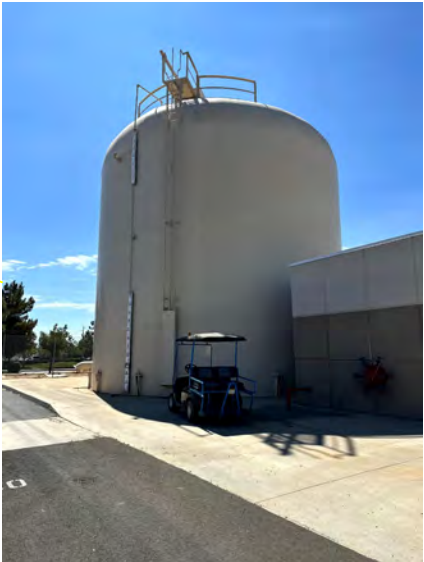
Water tank with backup power situated slightly south of the subject property
