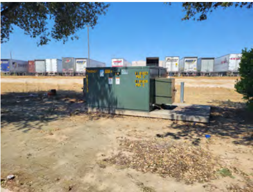
SCE Structure within the southeast portion of the subject property along Indian Ave
