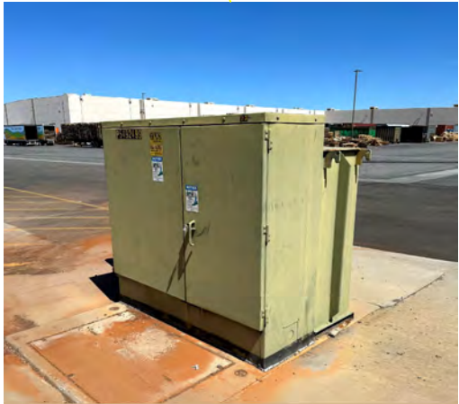
SCE Structure next to water tank outside of the southern portion of the subject property
