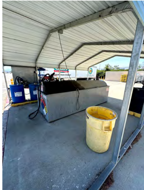
Diesel filling station and propane tank storage at southwest corner of the Lowe's Distribution Center
