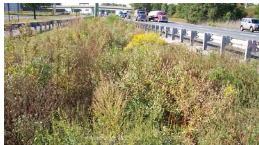
Bioretention facilities can provide food and shelter for potentially hazardous wildlife, but may be suitable with modification.
