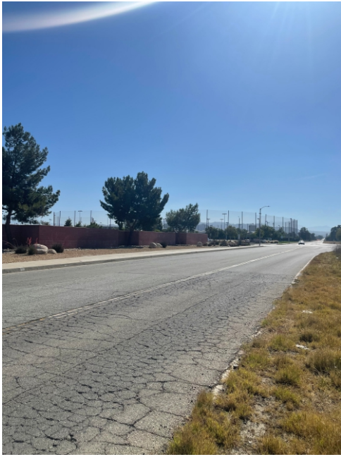
Photo 9: Northern Boundary of the Project Site Facing Northeast.
