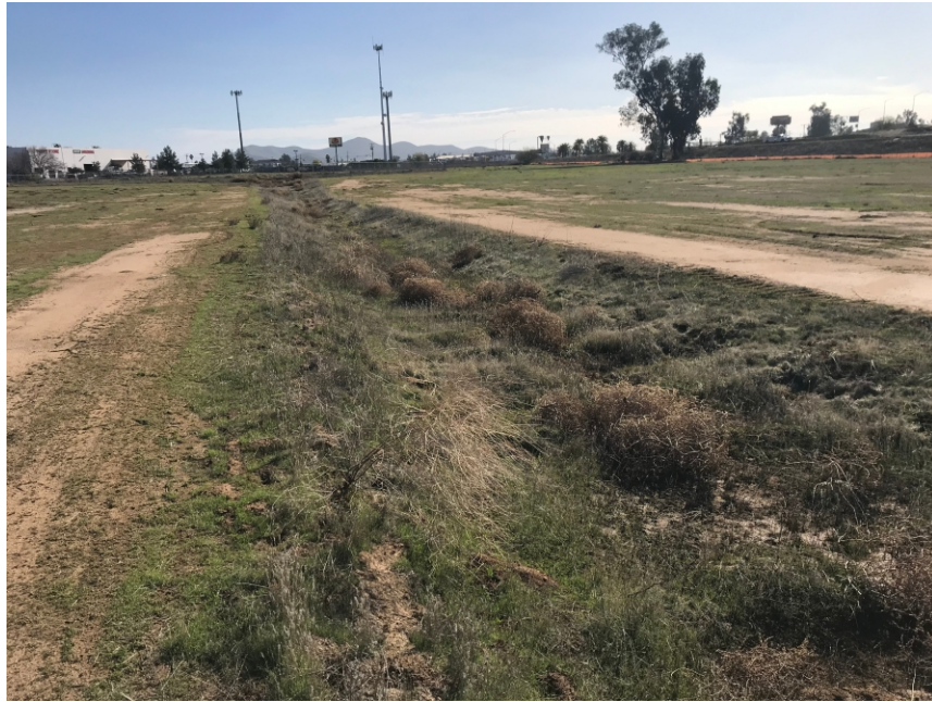
Photo 3: Abandoned Riverside County Flood Control Line B-Romoland Master Drainage Plan Facing Southeast.
