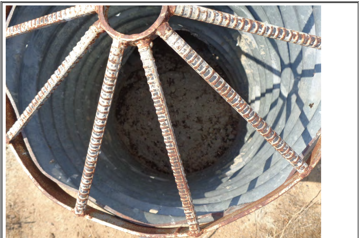
Photograph Number 14: Top view of drainpipe associated with the catch basin.
