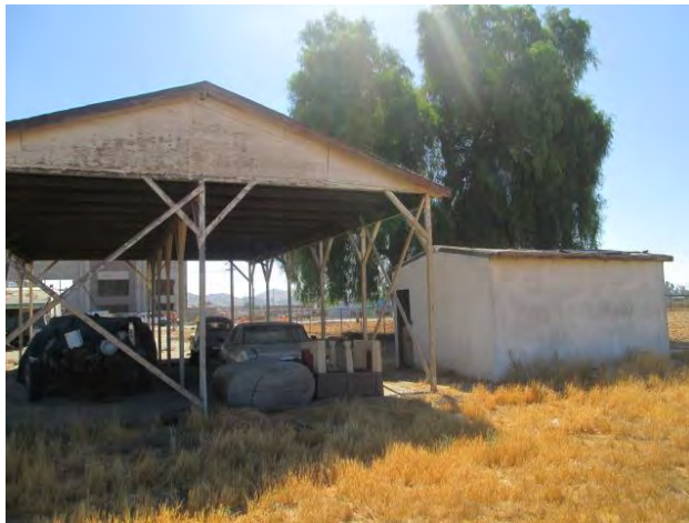
5. Carport/canopy and shed at 2980 Wilson Avenue.
