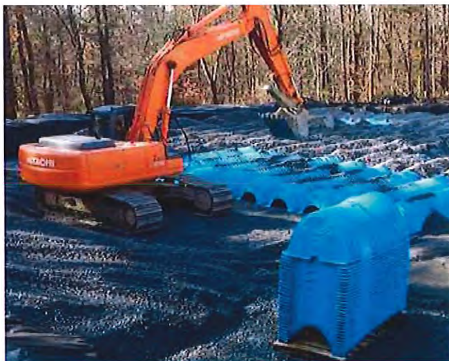
CULTEC CHAMBERS STACK ON SKIDS FOR EASY LOADING, UNLOADING AND STOCKPILING
