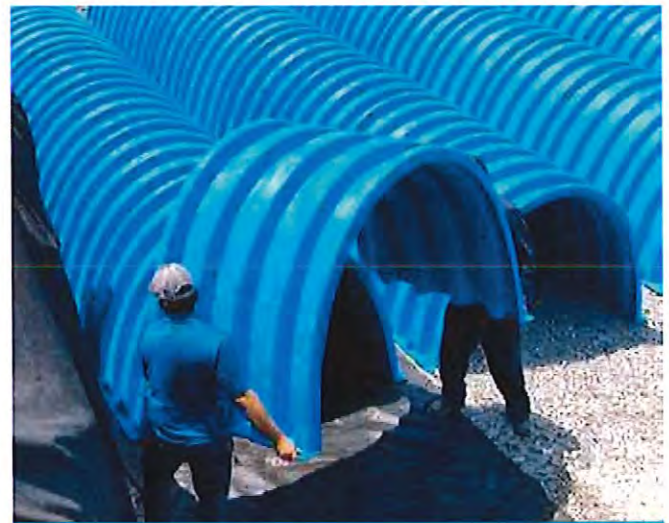
CULTEC CHAMBERS CAN BE HAND CARRIED FOR EASE OF INSTALLATION
