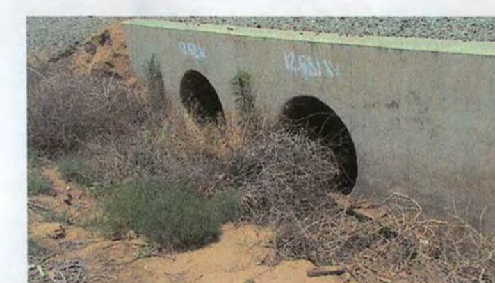
#13 - DOUBLE 36IN PIPE AT THE UPSTREAM END FACING EAST
