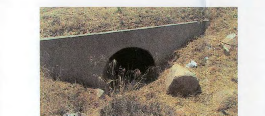
#19 - DOWNSTREAM END OF SINGLE 42IN PIPE CROSSING HARVILL AVE FACING SOUTHWEST
