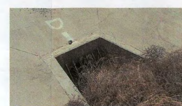
#22 - SINGLE 36IN PIPE AT HARVILL AVE AND OLEANDER AVE FACING SOUTH
