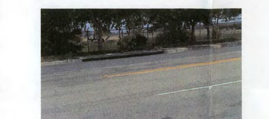
#23 - CATCH BASIN ON HARVILL AVE AND OLEANDER AVE FACING SOUTHEAST
