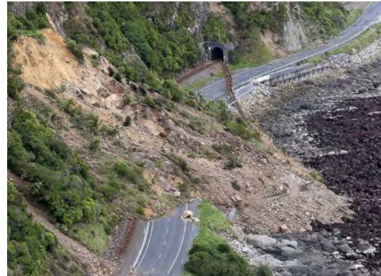
Examples of seismically induced ground failures include liquefaction (left photo) and landslides (right photo) from the 2011 M6.3 Christchurch, New Zealand Earthquake and the 2016 M7.8 Kaikoura, New Zealand Earthquake, respectively.
