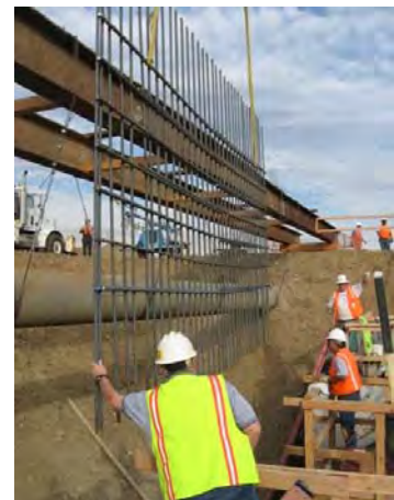
Metropolitan construction crews
