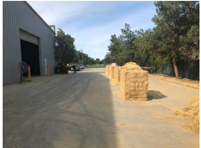
10. Northern portion of the Site facility.
