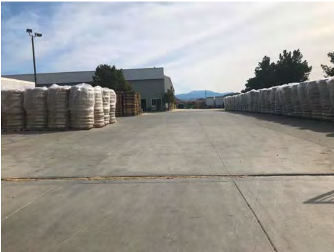
1. View east of the southern portion of the Site facility.
